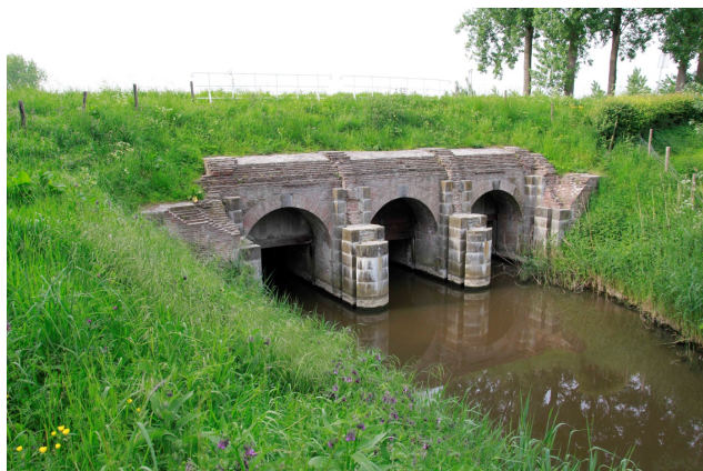
Figure 5. Land side of an inundation sluice, built in 1789 by the Estates General of the Dutch Republic at Zwartenhoek ( 51^{\circ}15'N and 3^{\circ}51'E ). Notice the double groove in the protruding parts in which beams could be installed. As the space in between the beams could be filled with earth, this construction was strong enough to prevent the fresh water from flowing seaward. After some weeks water in polders could reach a level of some decimetres. As soon as the threat of war disappeared, beams and earth were removed again (photo: Nellie de Kraker).
